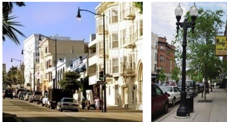
Figure (14) Lighting Posts for Vehicles and Pedestrians.
