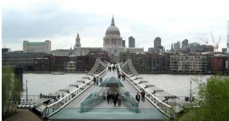
Figure (6) London Millennium Bridge
