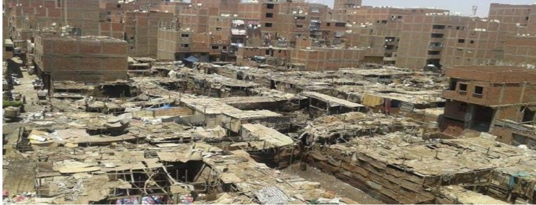
Figure 7. The Urban Degradation of Al-Zaraib Area.
